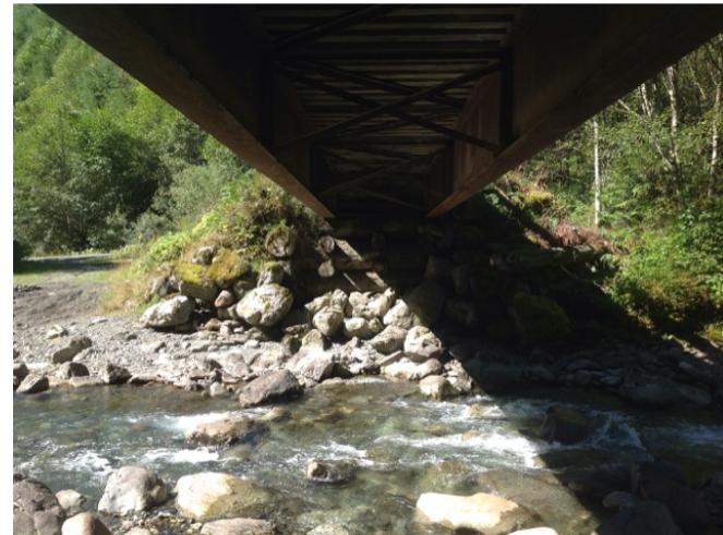
Right Bank Abutment when facing downstream
