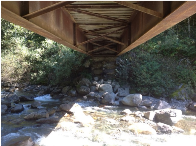
Left Bank Abutment when facing downstream
